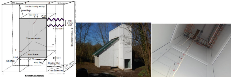
Fig. 6 The experimental structure for measuring airflow in relation to the rate of partial pressure change as a small portion of air passed over the cooling coils and the contained water vapor condensed. The cooling coils seen from looking up the right-hand column. How much air was cooled per second depended on the rate of condensation and the resulting airflow. With no condensation there was no measurable airflow, even though the air at the cooling coils showed a temperature reduction of 10 °C and a gain in density of 0.05 kg/m 3 . (©Peter Bunyard 2024)
